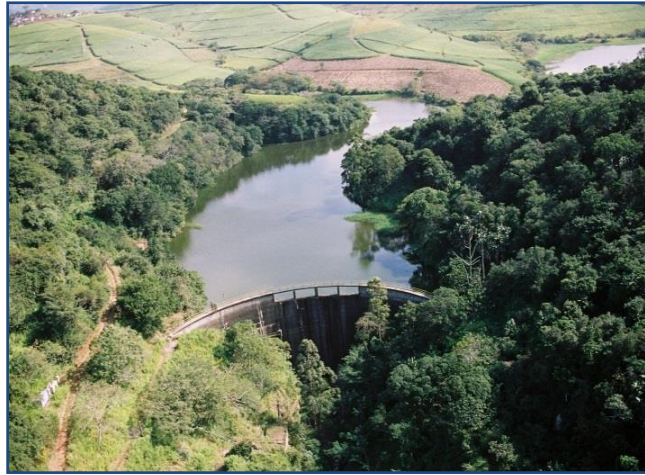
Figure 11.20 E.J. Smith Dam.
