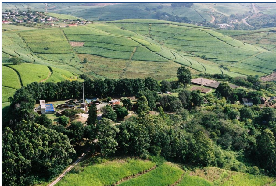
Figure 11.28 Umzinto Water Treatment Plant.
