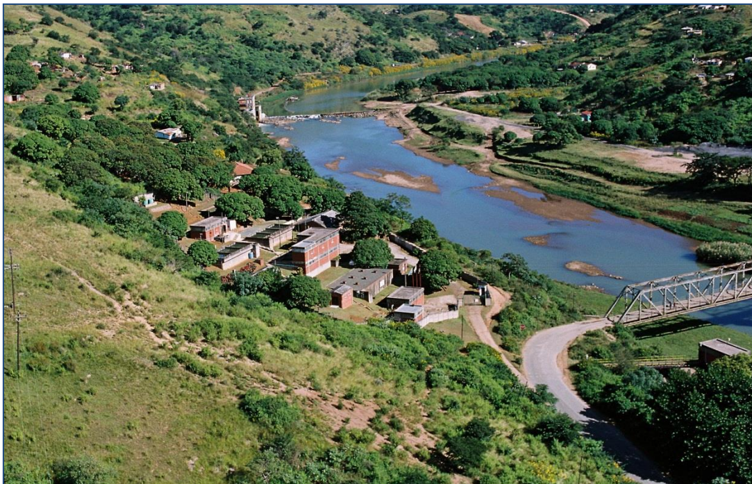
Figure 11.27 Craigieburn Water Treatment Plant (decommissioned).
