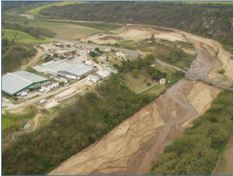
Figure 11.30 Mtwalume Water Treatment Plant.
