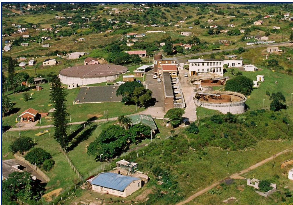
Figure 11.25 Amanzimtoti Water Treatment Plant.
