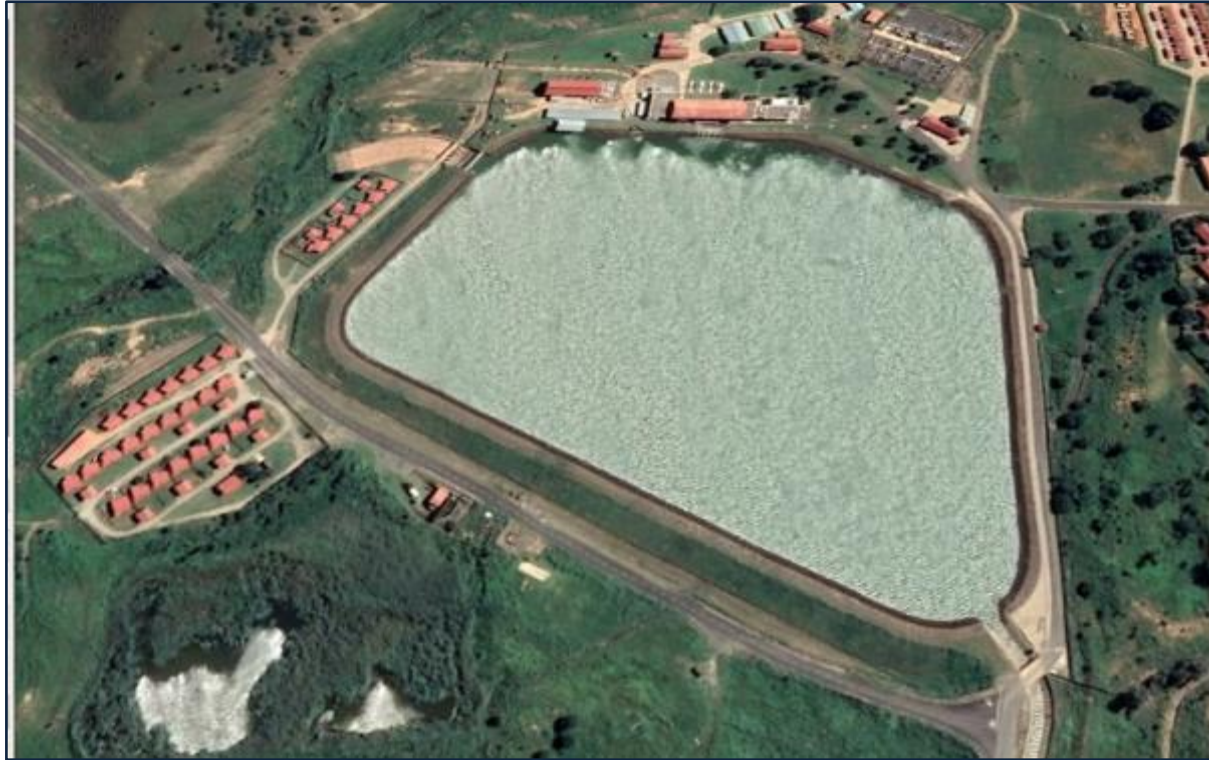
Figure 13.16 Jagersrust Balancing Dam (Google Earth 2019: website).
