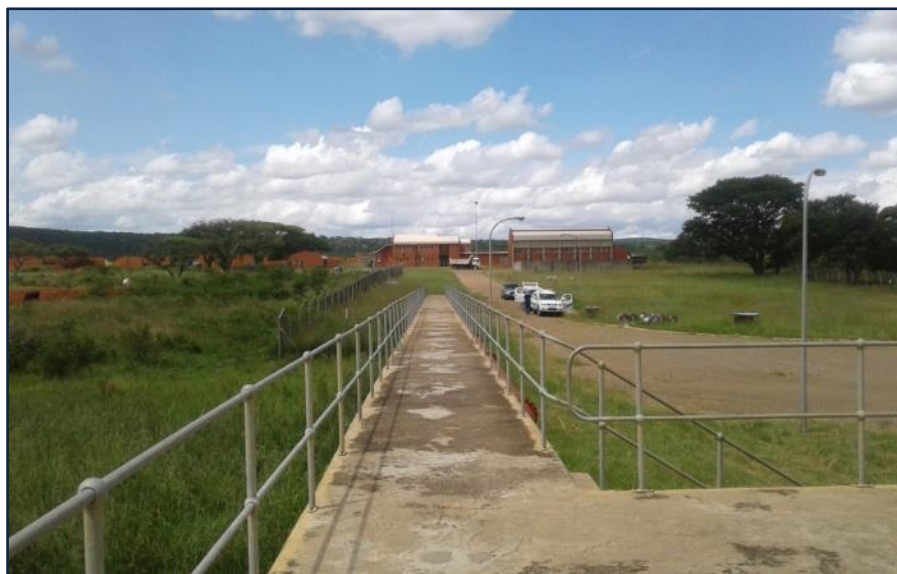
Figure 13.38 Olifantskop Water Treatment Plant (unknown date).
