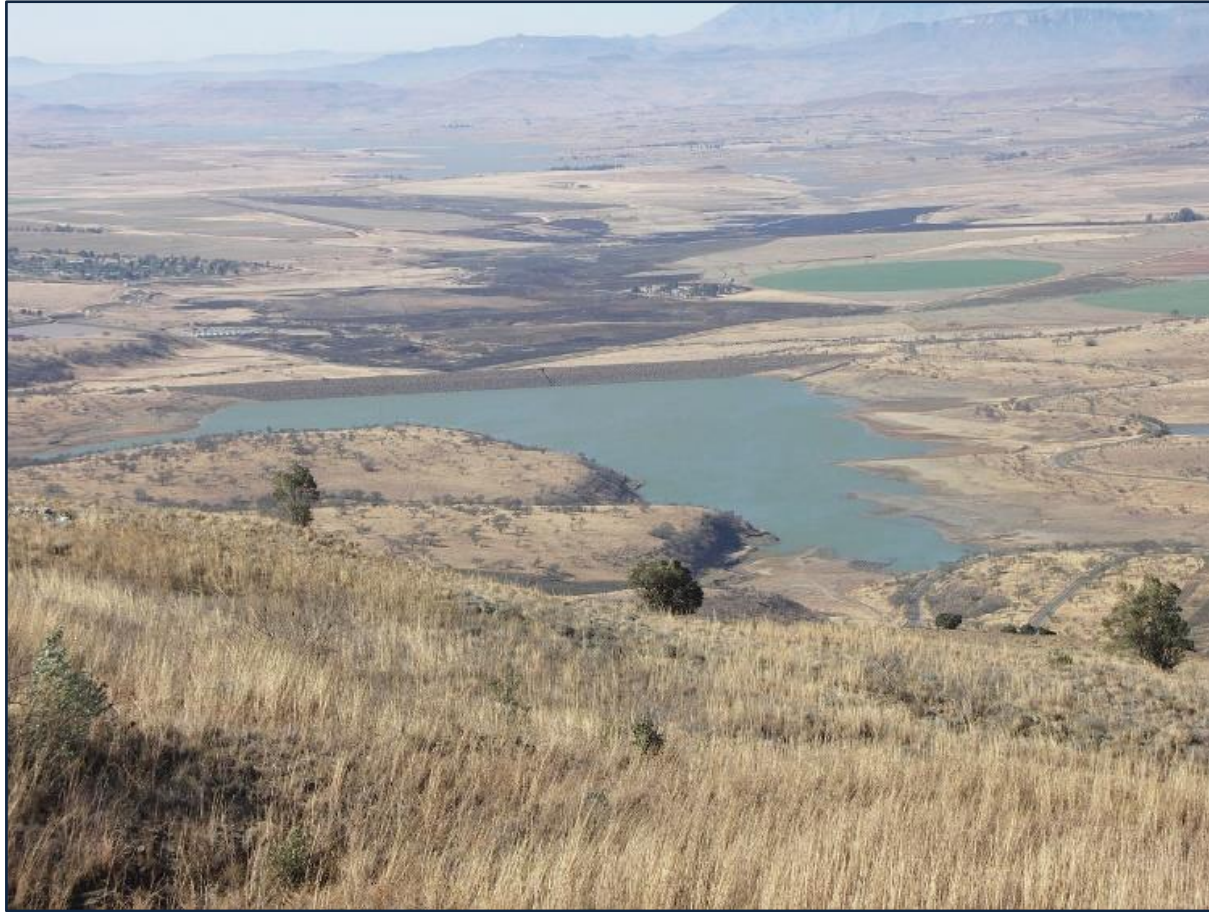
Figure 13.15 Kilburn Dam (DWS 2008: DWS website).
