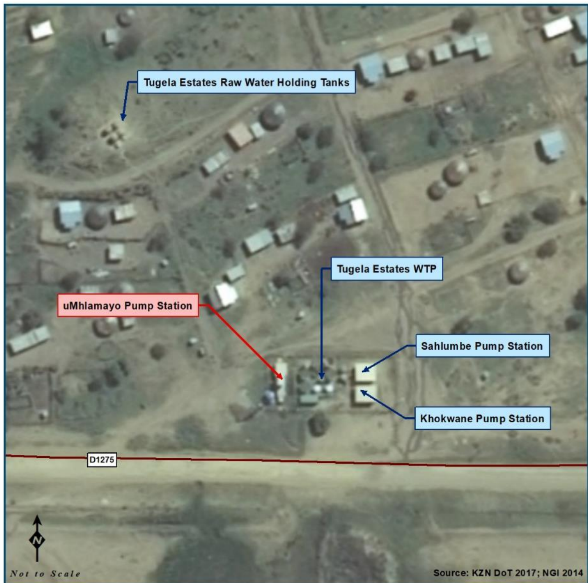
Figure 13.30 uMhlamayo Pump Station adjacent to the Tugela Estates WTP (KZN DoT 2017; NGI 2014).
