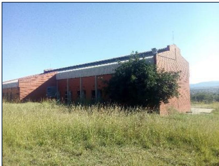
Figure 13.45 Petronella Reservoir Pump Station (Umgeni Water 2019).
