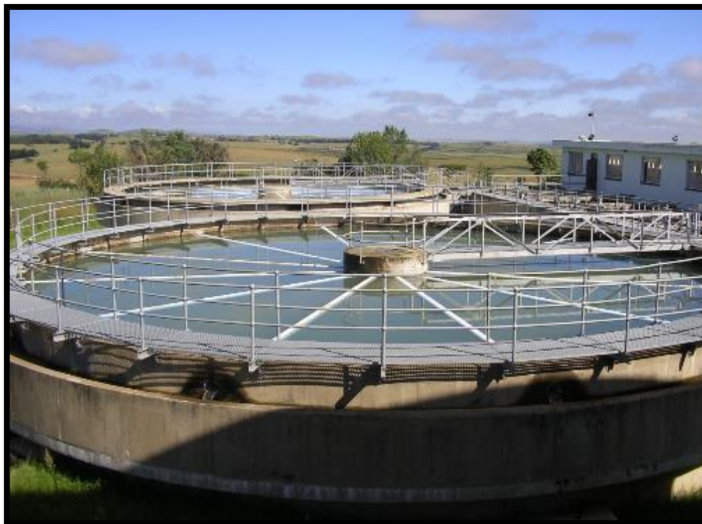
Figure 13.64 George Cross Water Treatment Plant (Bigen Africa, O & Manual, 2009)
