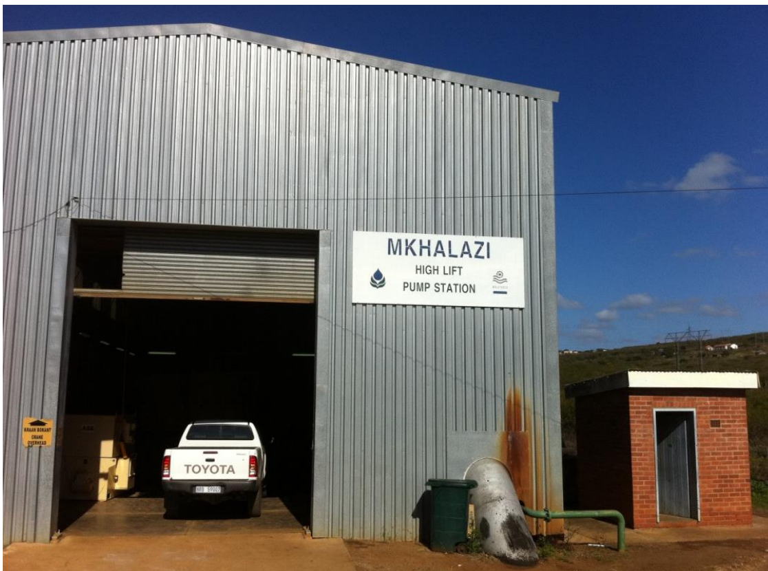
Figure 16.16 The Mkhhalazi High Lift Pump Station.
