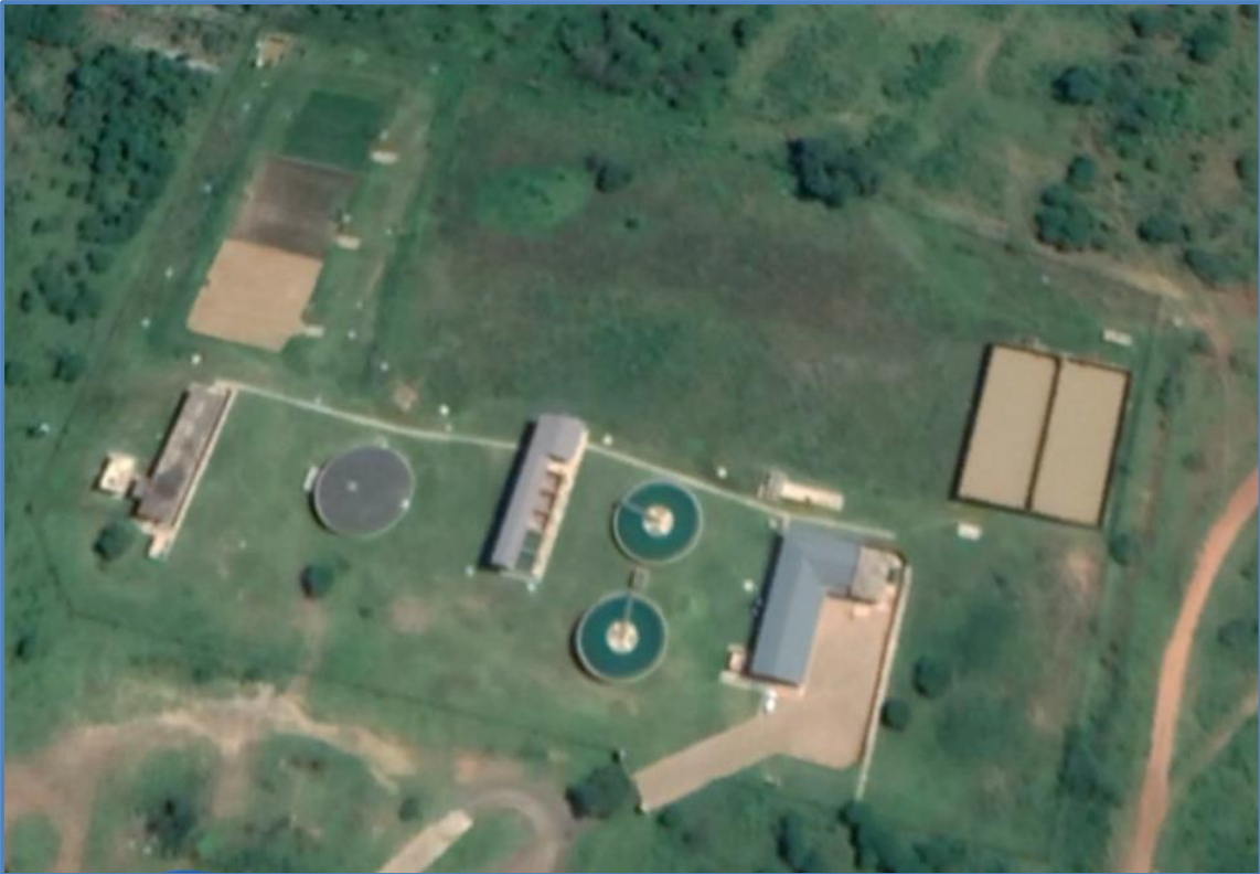
Figure 16.13 An aerial photo of the Middledrift WTP.
