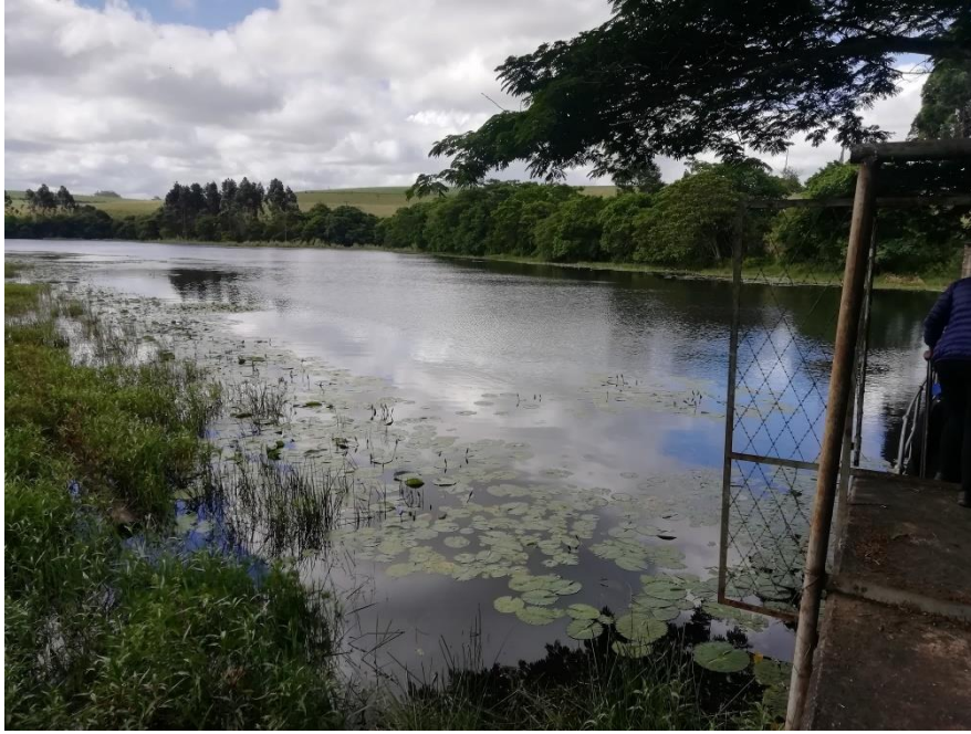
Figure 16.6 Rutledge Park Dam on 09 th November 2021 (Source: Umgeni Water).
