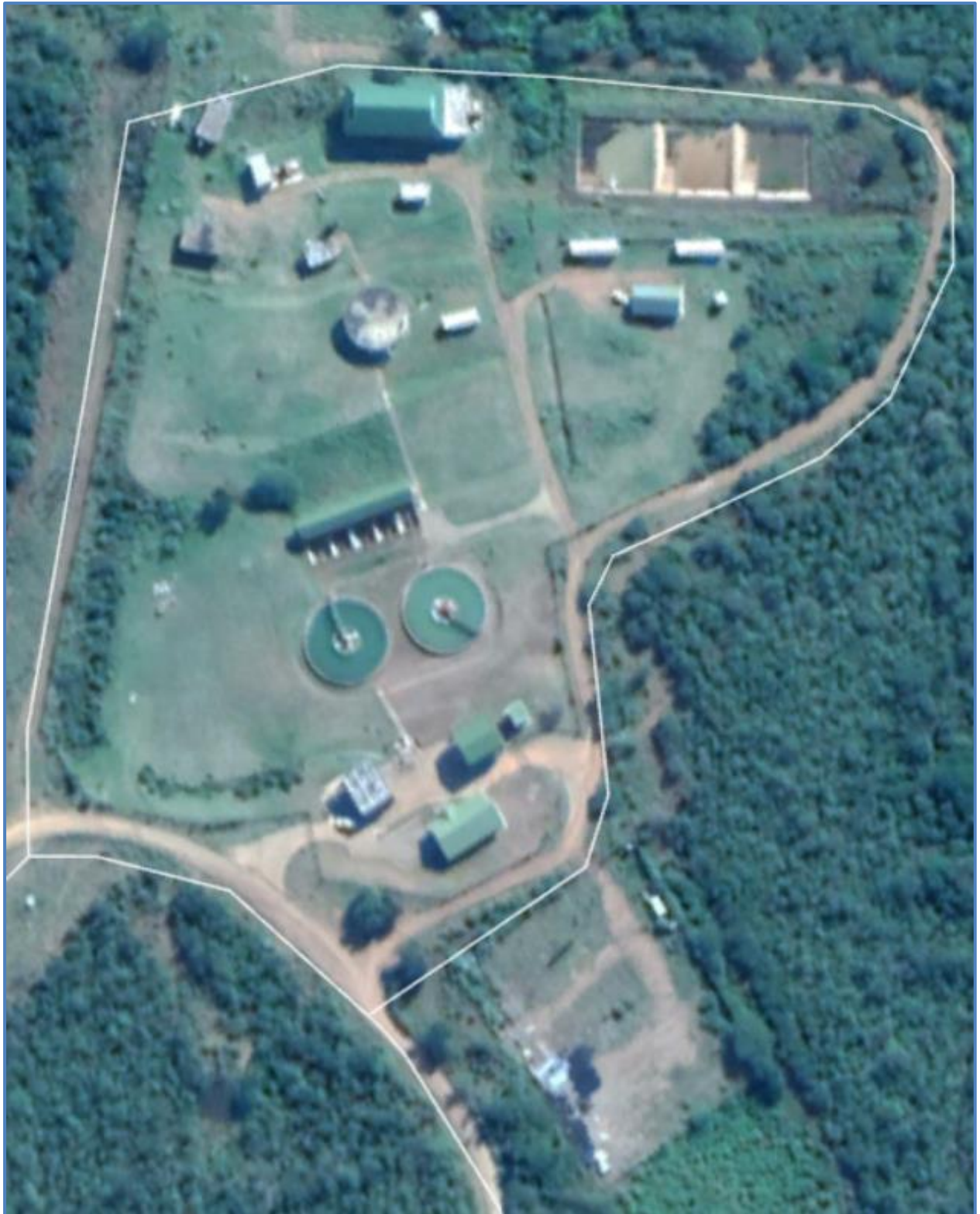
Figure 16.18 Greater Mthonjaneni WTP.
