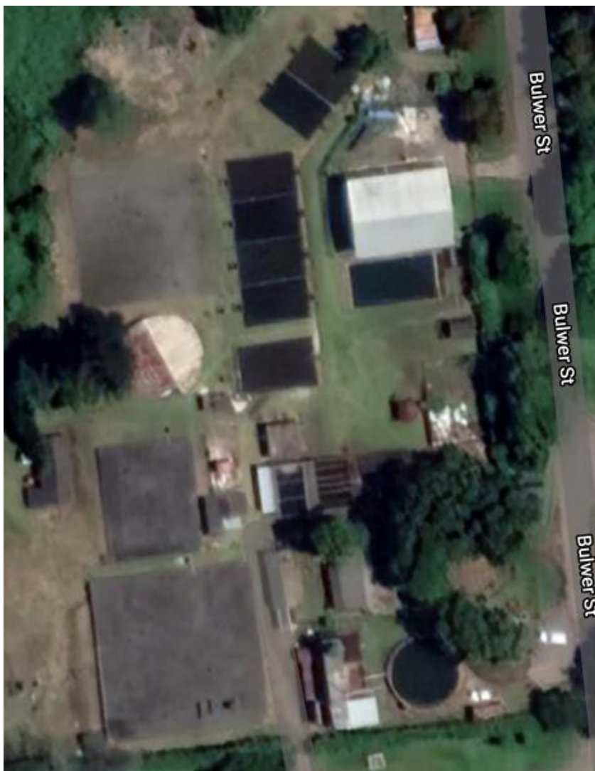
Figure 16.20 The Eshowe WTP.
