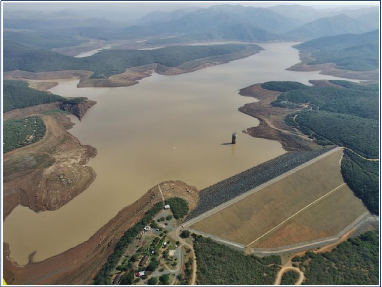
Figure 16.4 Goedertrouw Dam (Aerial photograph taken by Helene Smith showing the extent of the drop in water levels).
