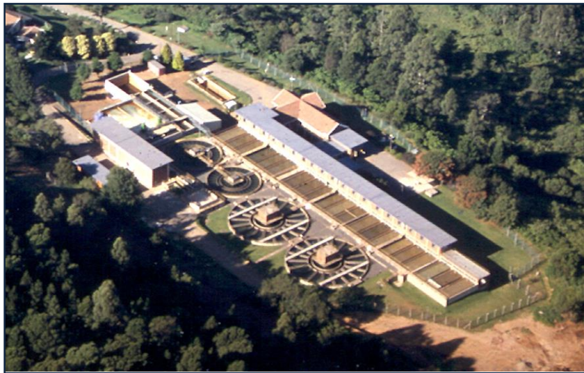
Figure 7.35 D.V. Harris Water Treatment Plant.
