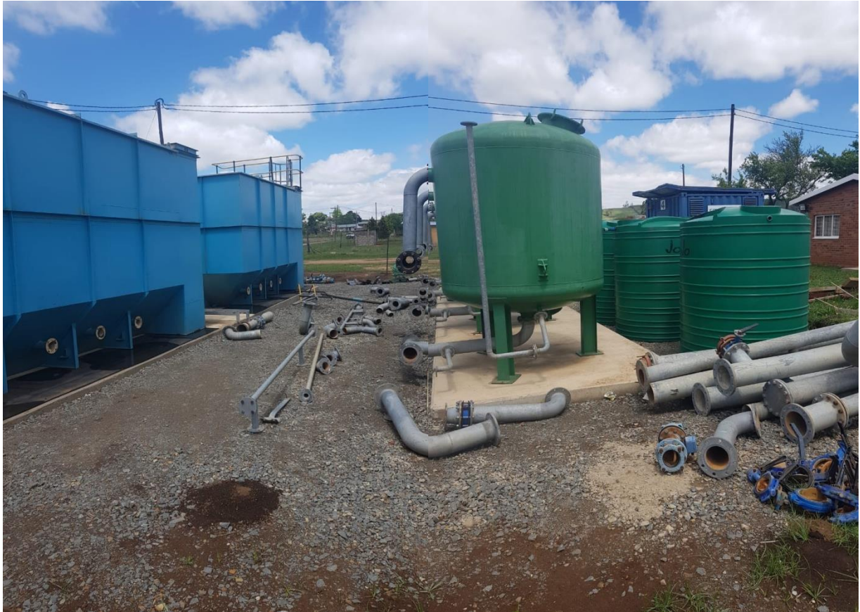
Figure 7.80 1 MI/day being constructed at the Lidgetton System.
