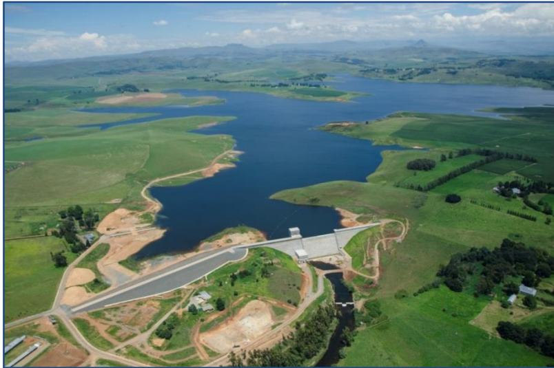
Figure 7.26 Spring Grove Dam.
