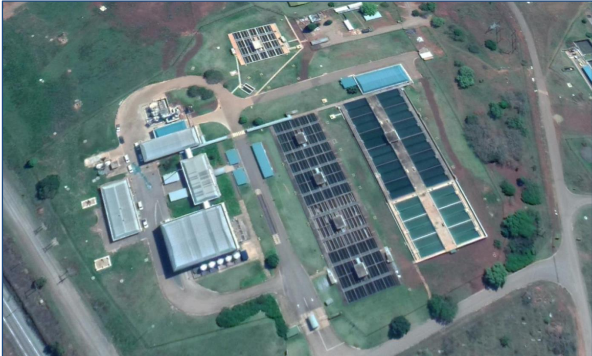
Figure 7.29 Midmar Water Treatment Plant after the upgrade.
