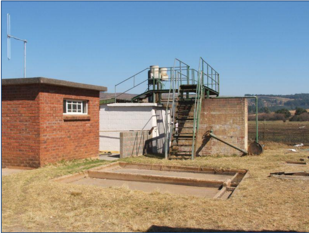
Figure 7.78 Lidgetton WTP sand wash bays with old dosing system (uMgungundlovu District Municipality 2010)
