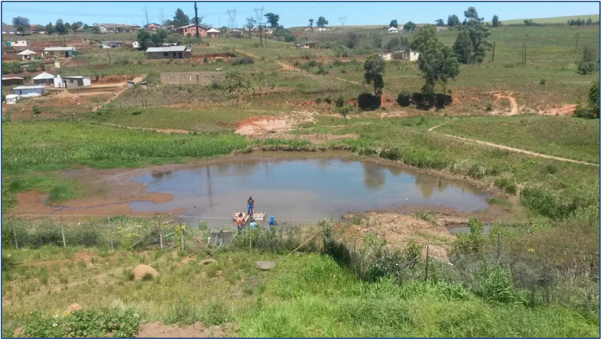
Figure 7.74 Dam supplying Appelsbosch WTP (Umgeni Water 2015).
