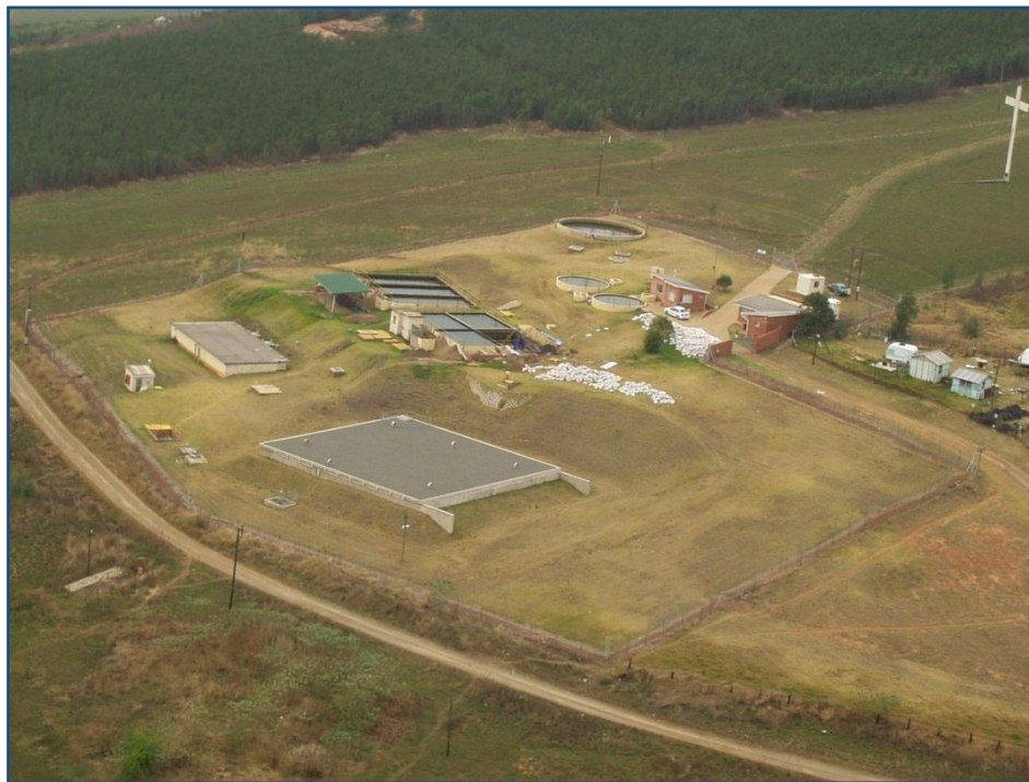
Figure 8.5 Ixopo Water Treatment Plant.
