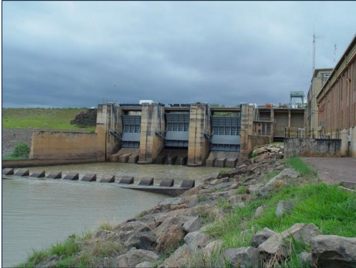
Figure 13.18 Driel Barrage Dam (DWS unknown date: DWS website).
