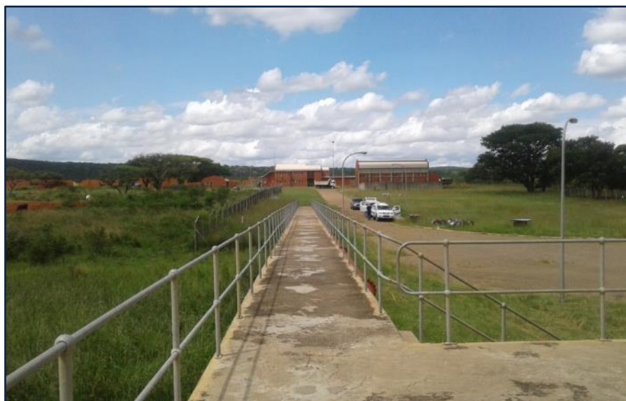
Figure 13.38 Olifantskop Water Treatment Plant (unknown date).
