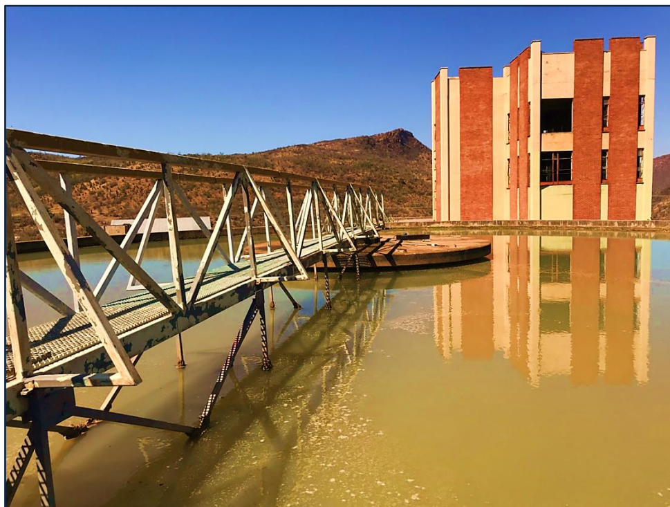
Figure 13.24 Ezakheni Water Treatment Plant (unknown date).
