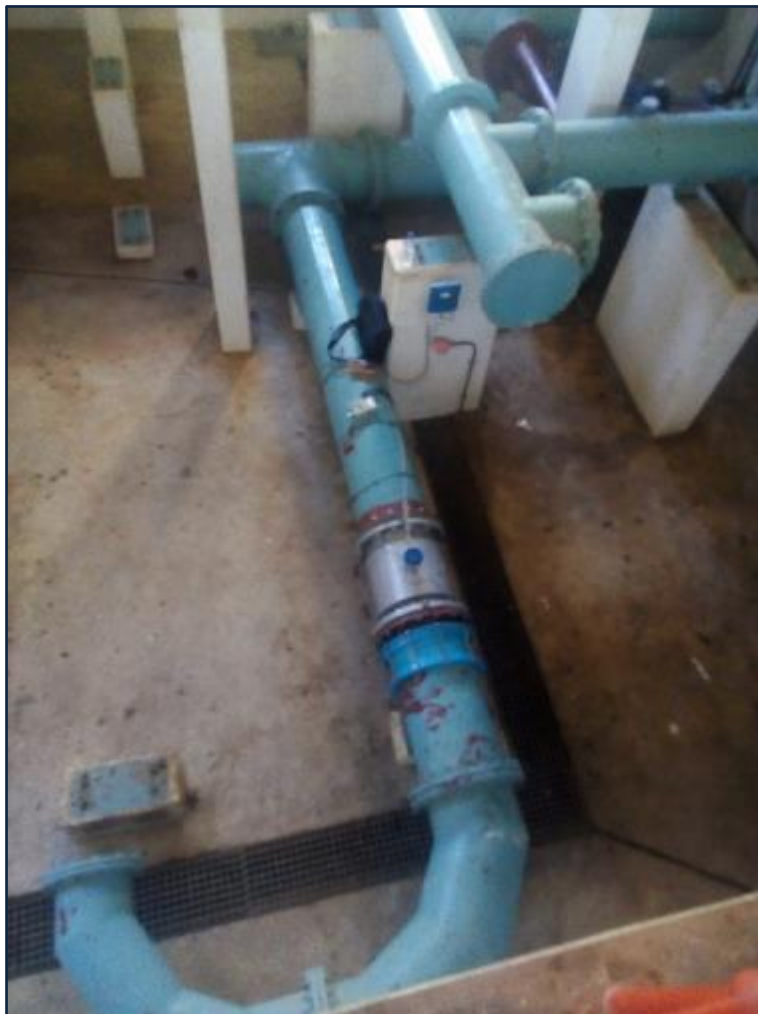
Figure 13.47 Ekuvukeni sales meter (Umgeni Water 2019).
