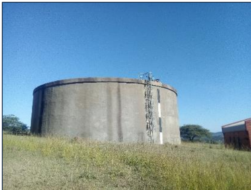
Figure 13.43 Petronella Reservoir (Umgeni Water 2019).
