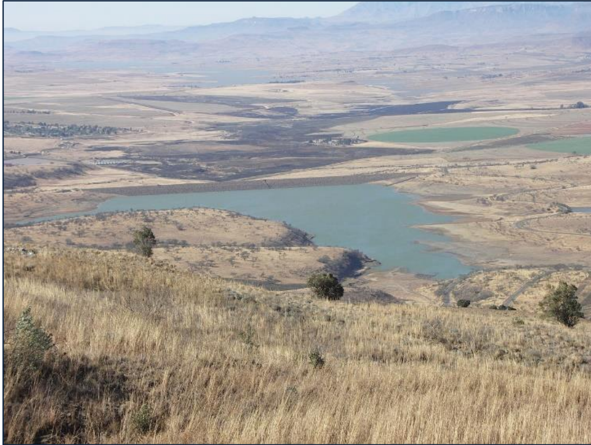
Figure 13.15 Kilburn Dam (DWS 2008: DWS website).
