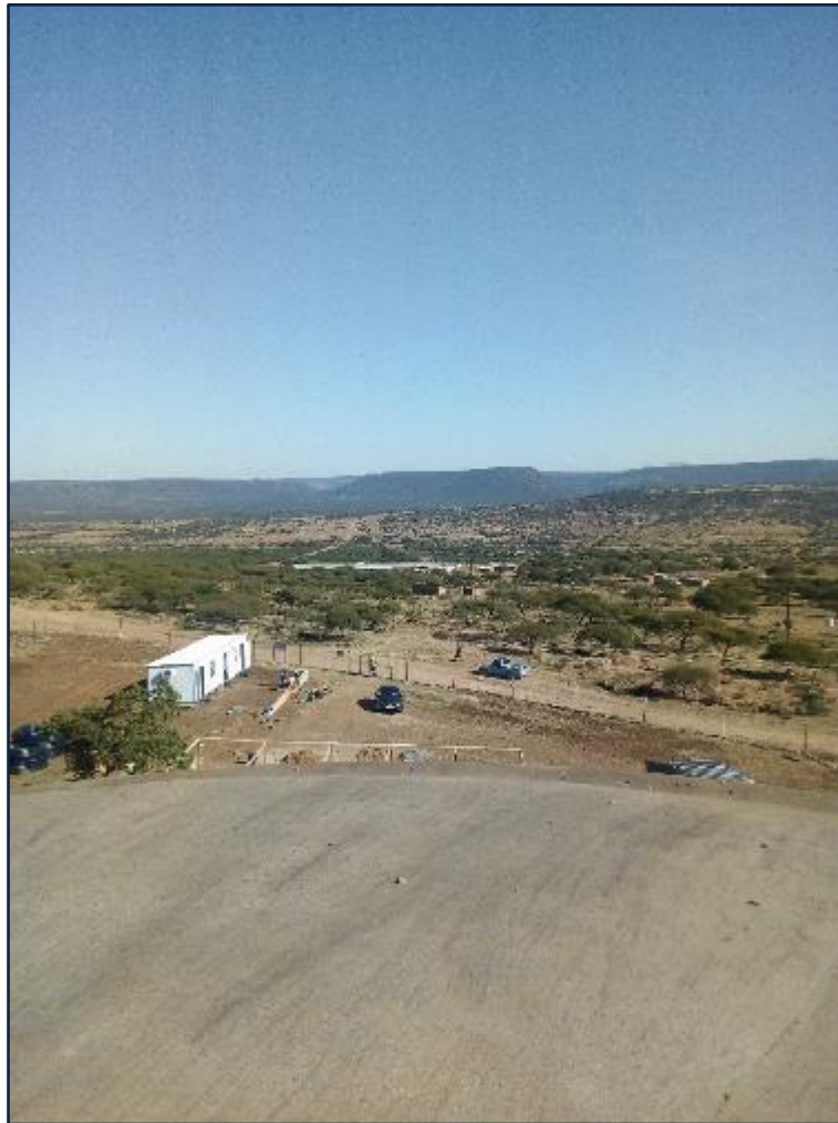
Figure 13.44 Pipeline servitude from Petronella Reservoir (Umgeni Water 2019).
