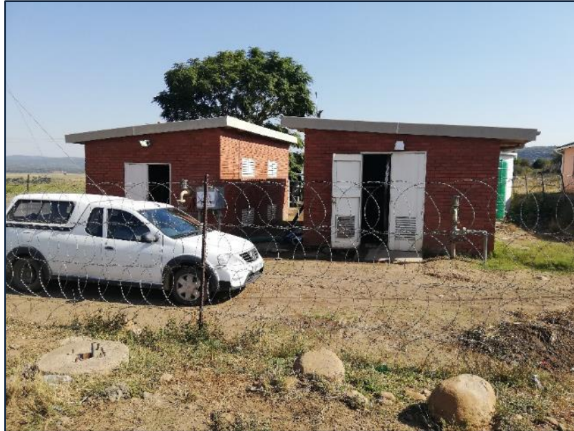
Figure 13.35 Khokwane Pump Station and Sahlumbe Pump Station on the Tugela Estates WTP site (Umgeni Water 2019).
