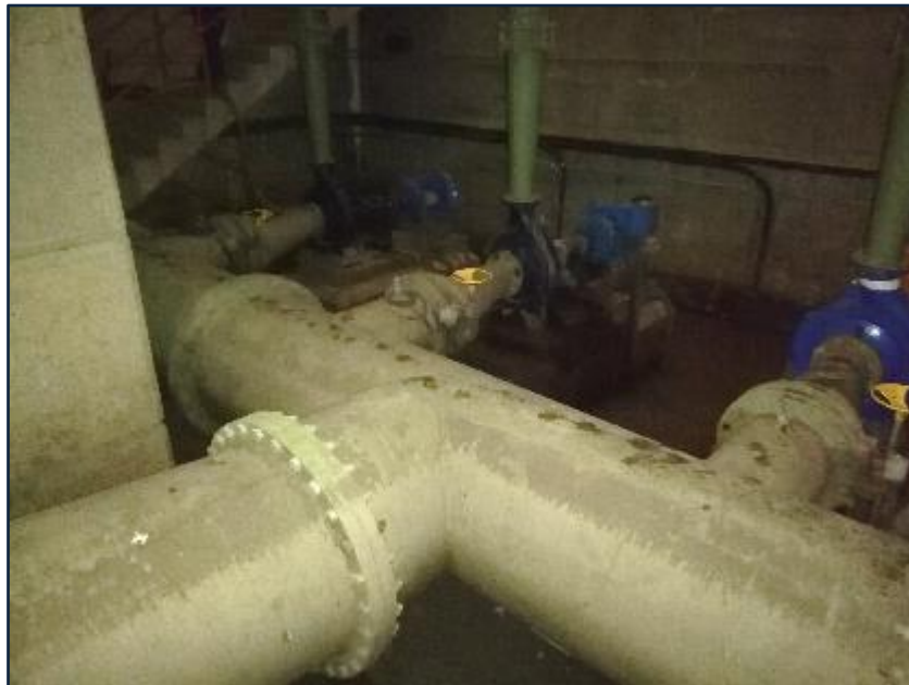
Figure 13.41 Olifantskop raw water pumps (Umgeni Water 2019).
