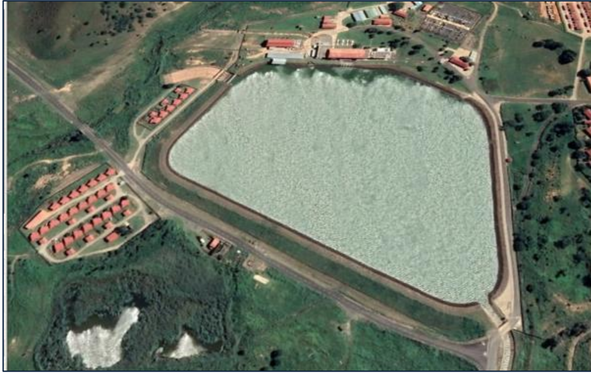
Figure 13.16 Jagersrust Balancing Dam (Google Earth 2019: website).
