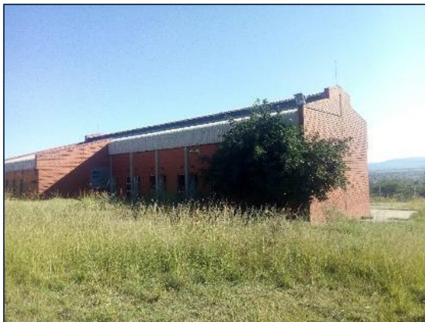
Figure 13.45 Petronella Reservoir Pump Station (Umgeni Water 2019).
