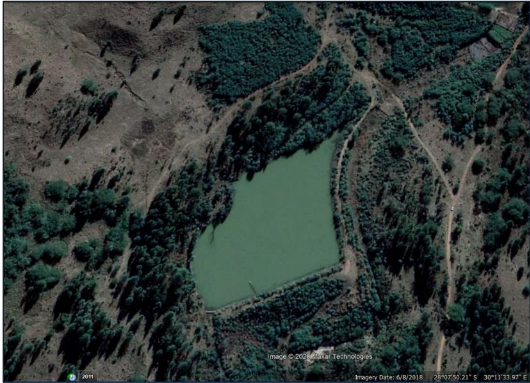
Figure 14.17 Lower Mpaté Dam (Google Earth 2018: website).
