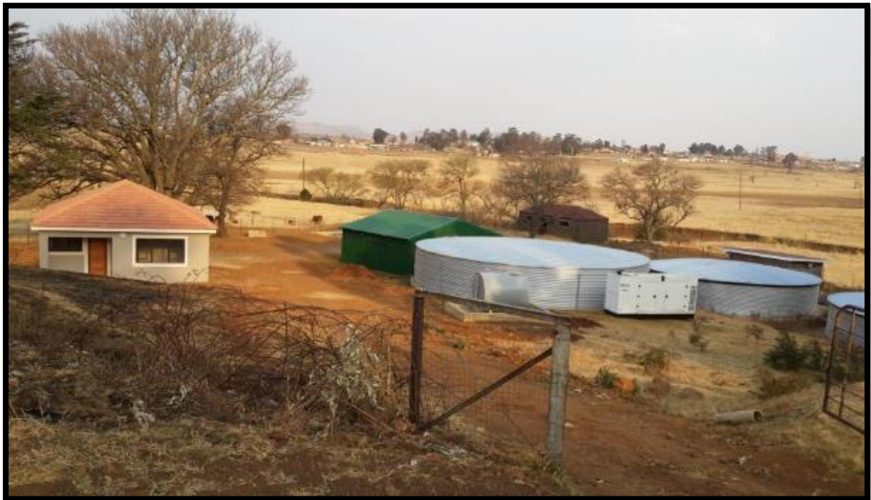
Figure 14.43 Photo of Charlestown Water Treatment Plant (July 2018).
