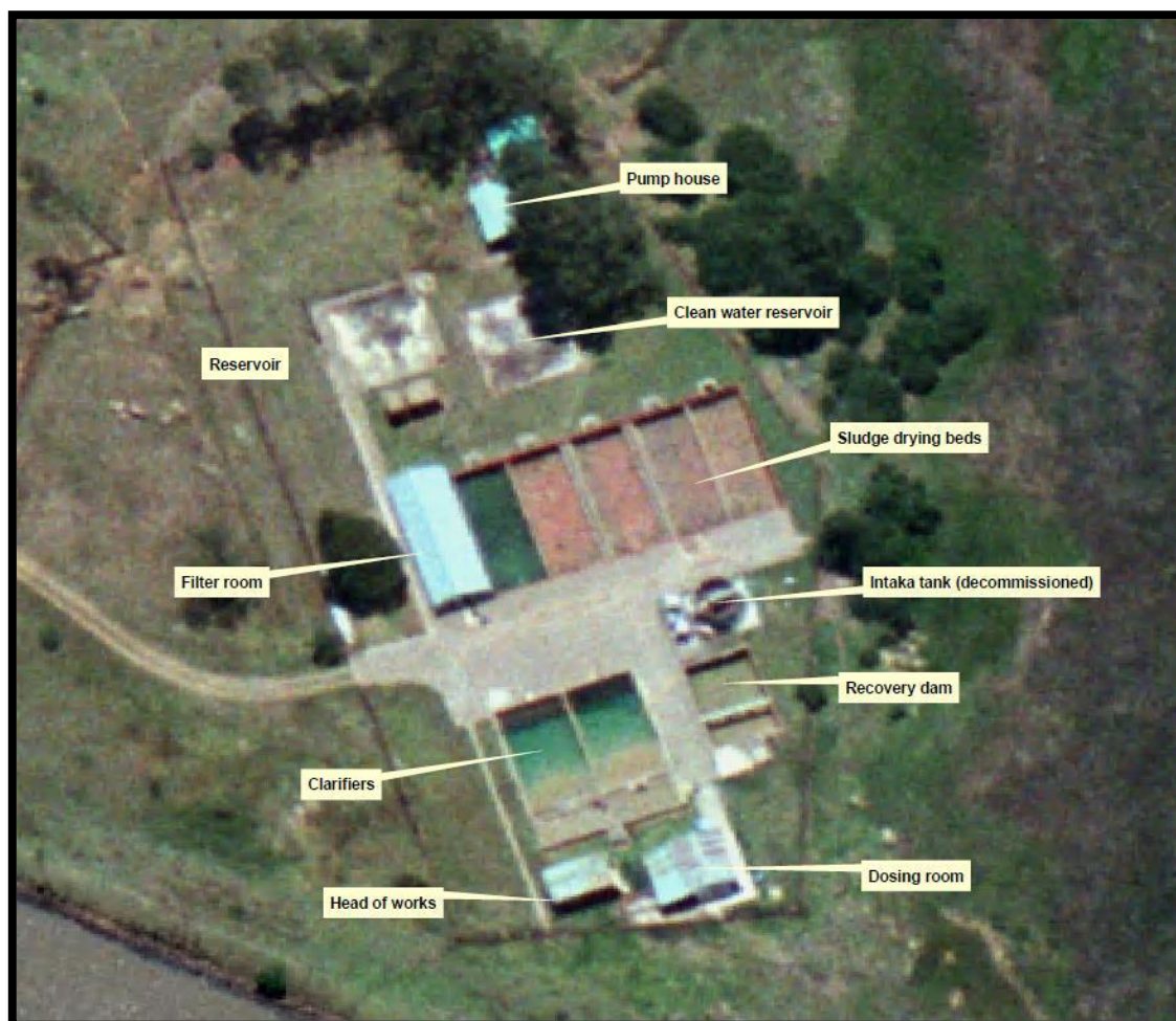
Figure 14.31 Aerial Image of Dannhauser Water Treatment Plant (ADM O&M Manual May 2016)
