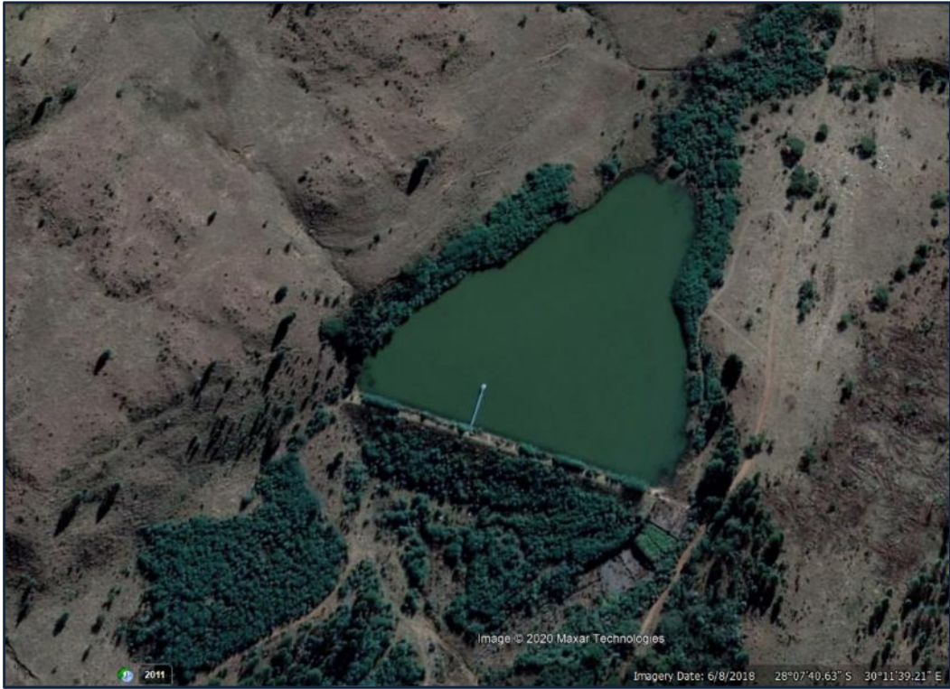
Figure 14.16 Upper Mpate Dam (Google Earth 2018: website).
