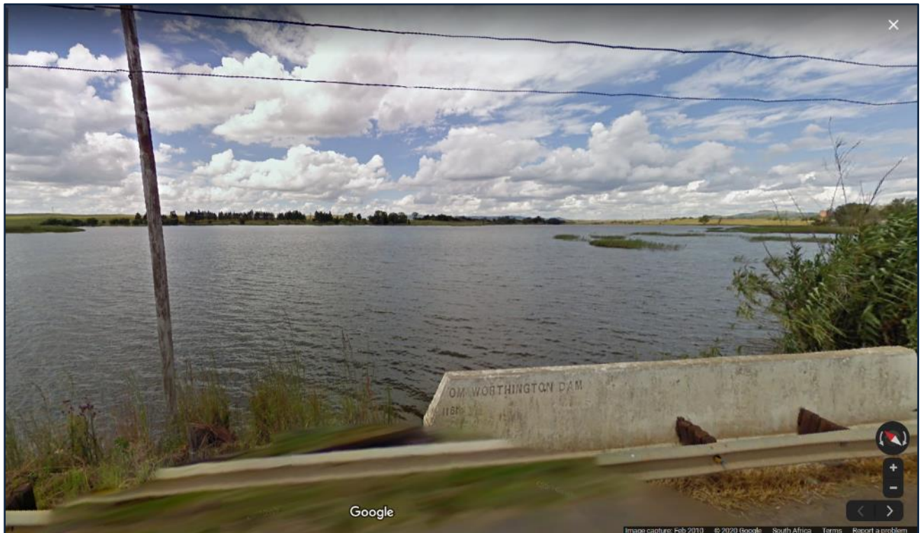
Figure 14.12 Tom Worthington Dam (Google StreetView 2010: website).
