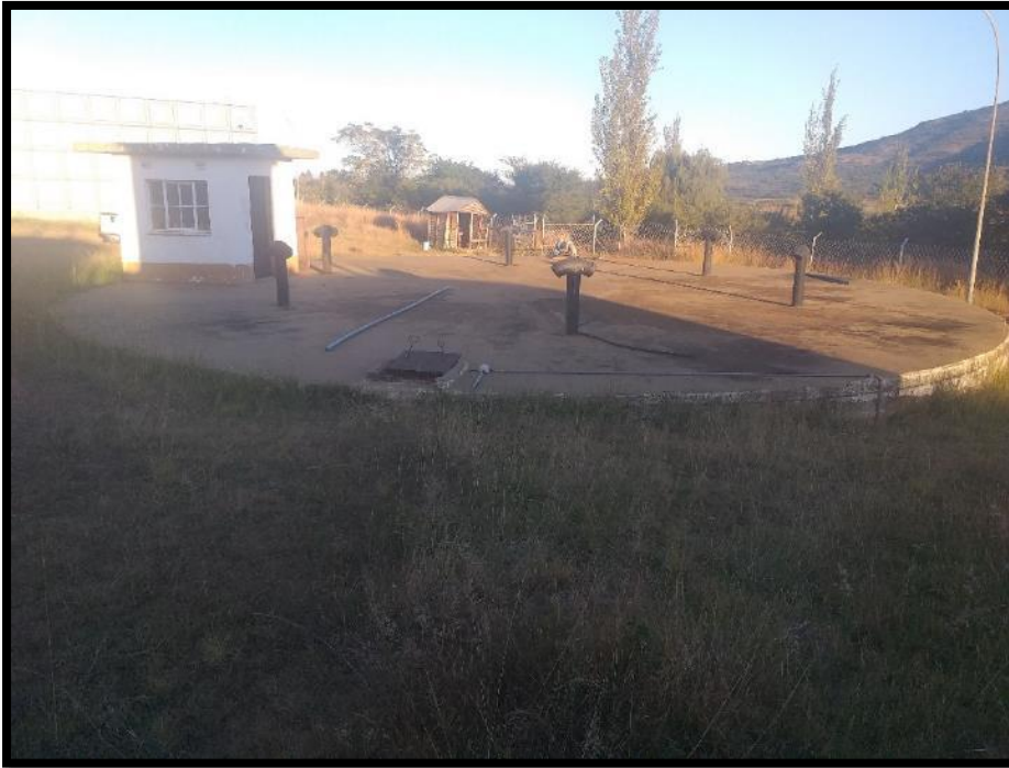
Figure 14.42 Utrecht Clear water Reservoir
