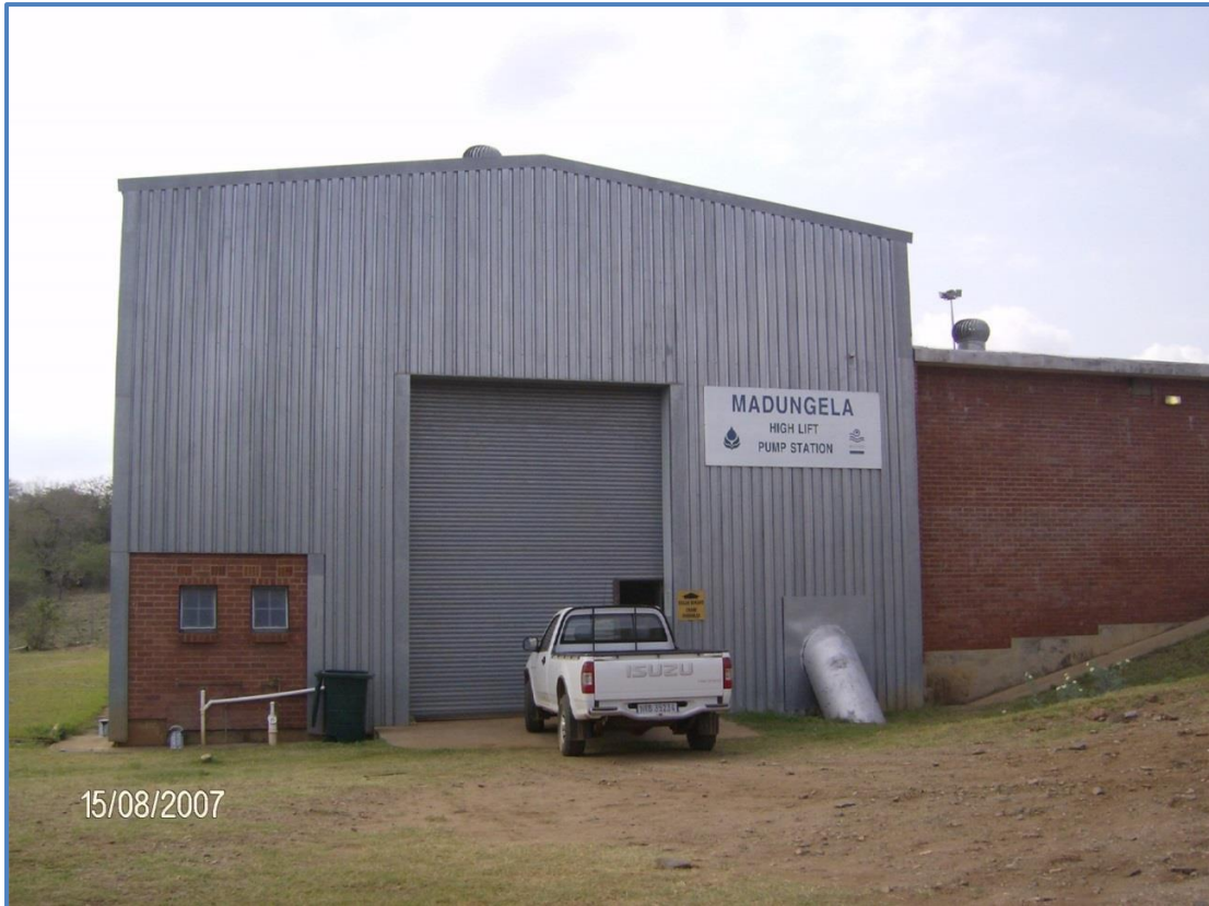
Figure 16.14 Madungela High Lift Pump Station
