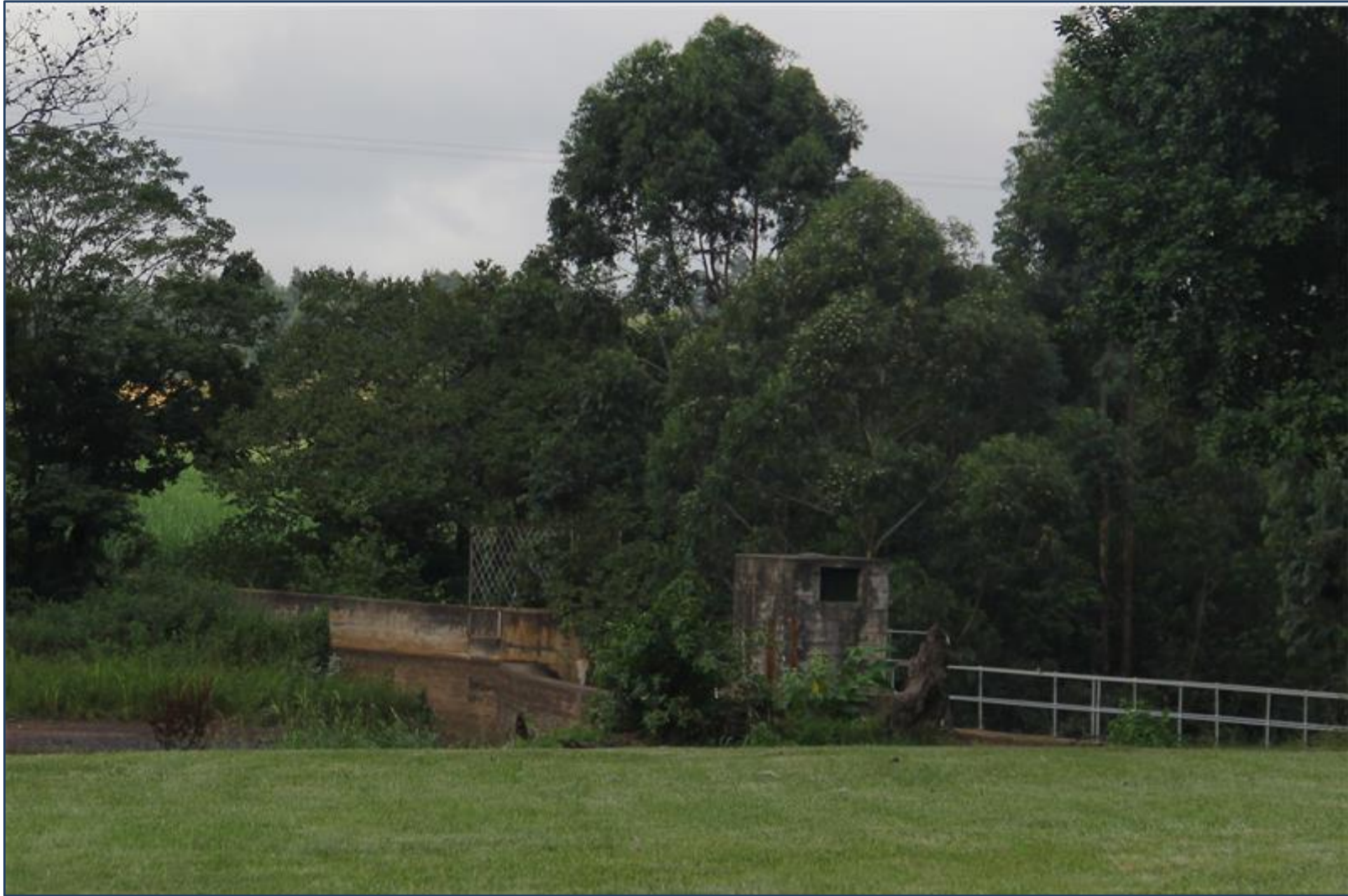
Figure 16.6 Rutledge Park Dam (Zululand Observer 2016: website).
