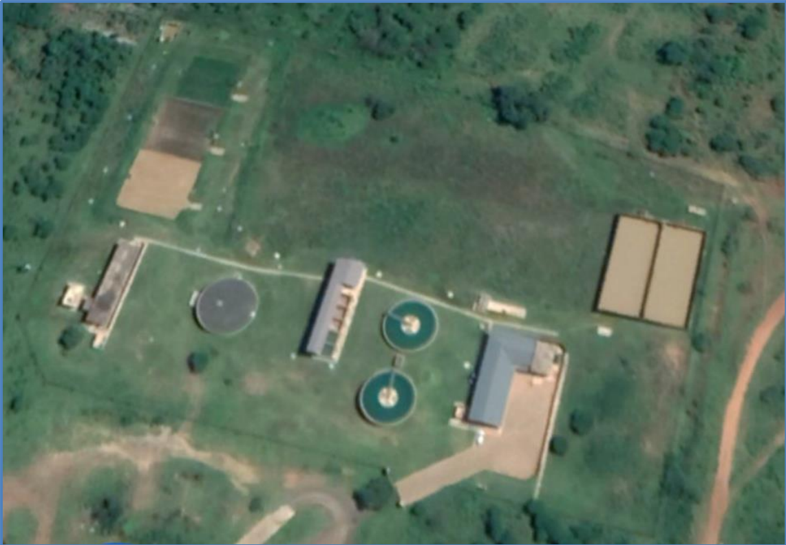
Figure 16.12 Aerial Photo of Middledrift WTP
