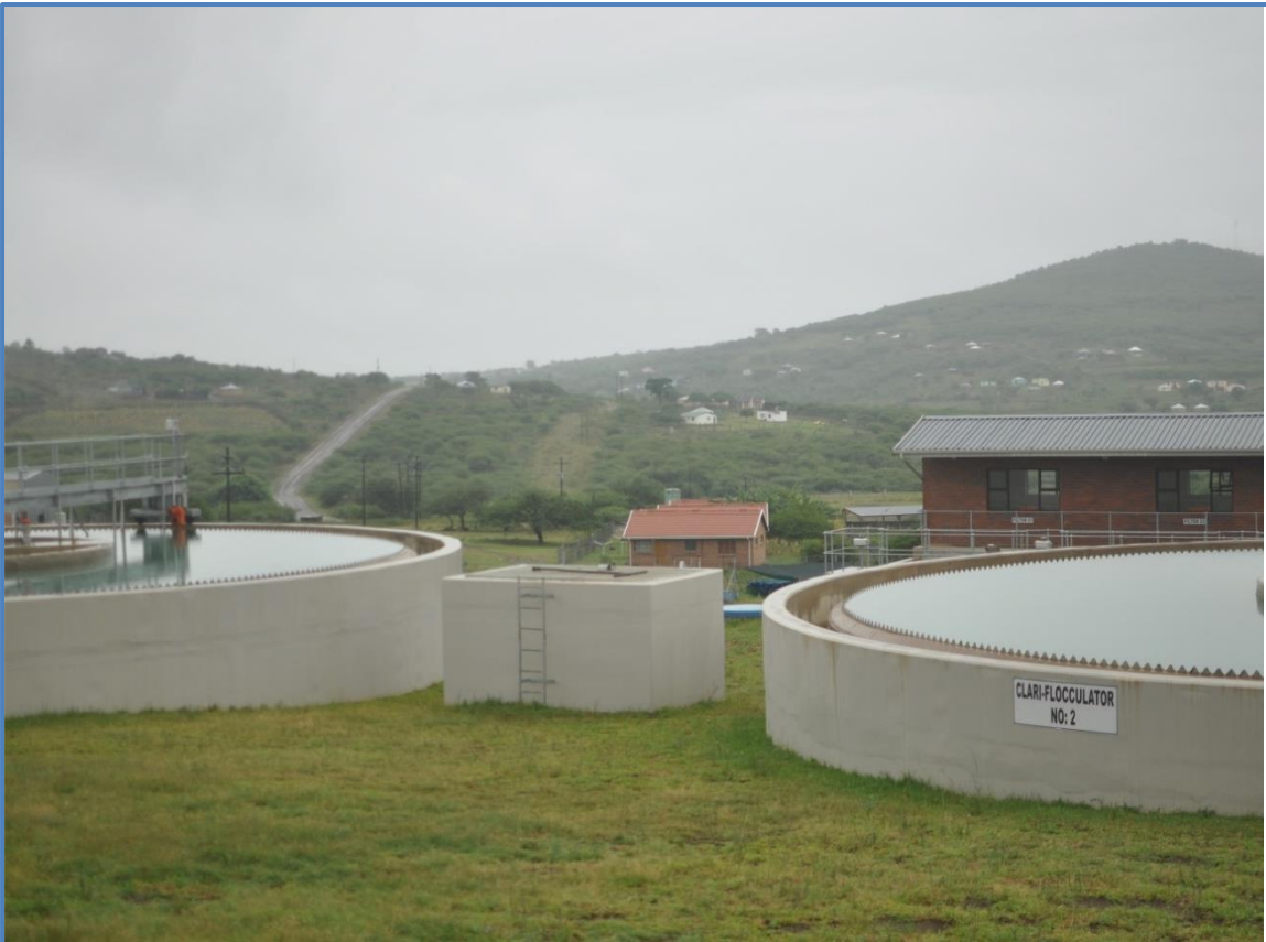
Figure 16.13 Photo of Middledrift WTP Clarifiers
