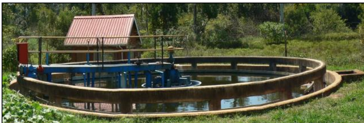
Figure 19.38 Richmond WWW clarifier.
