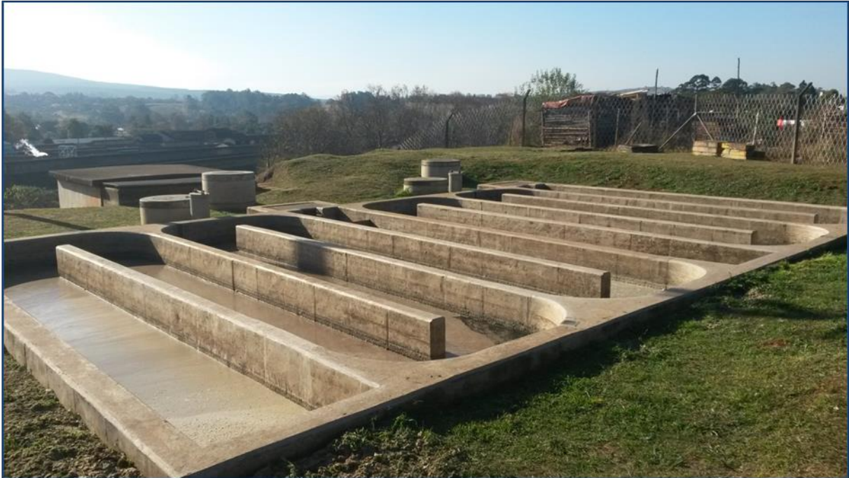
Figure 19.14 Howick WWT Chlorine Contact Tank.
