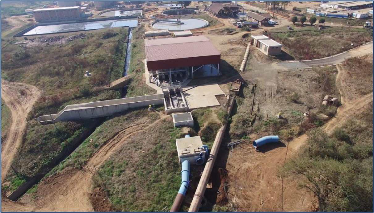
Figure 19.43 New head of works in the foreground with overflow channel teeing-off to the left.
