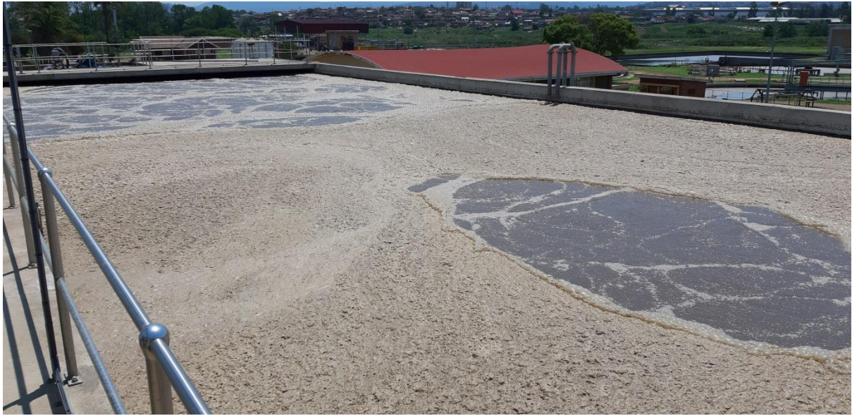
Figure 19.7 Darvill Aeration Basin.
