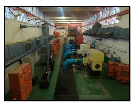
Figure 14.23 Photo of High Lift Pump Station at Ngagane WTP (May 2020)
