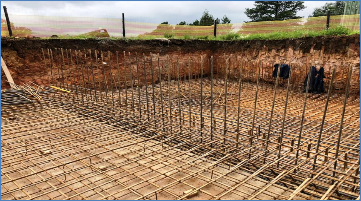
Figure.12.54 Transfer Pump Station in Construction (Late 2019)
