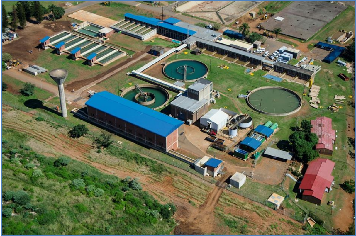
Figure 12.17 Hazelmere Water Treatment Plant.
